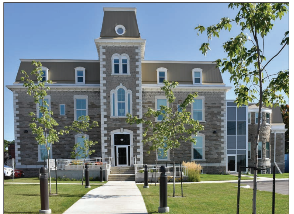
Newly landscaped exterior after demolition of the 1960s chancery office.
